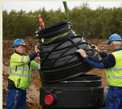
Installing the Tegra 1000 cone.
